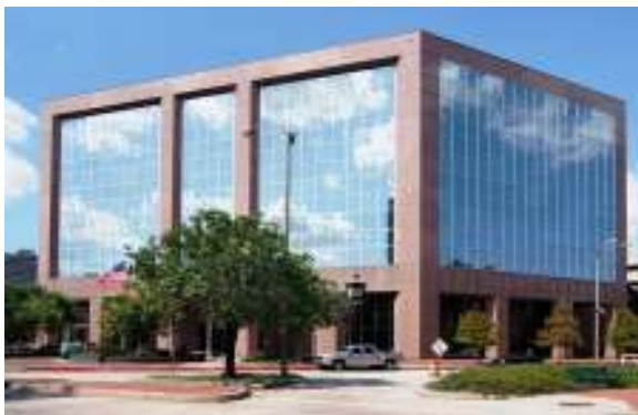
FRONT VIEW OF I CITY PLAZA DOWNTOWN BATON ROUGE
